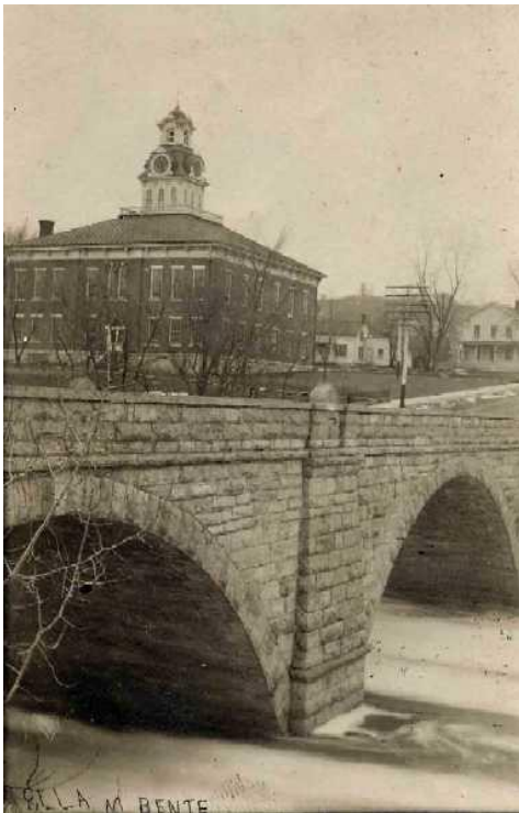
Clayton County Courthouse and Keystone arch bridge over Turkey River, ca 1911 (IA GenWeb Project, 2018)
